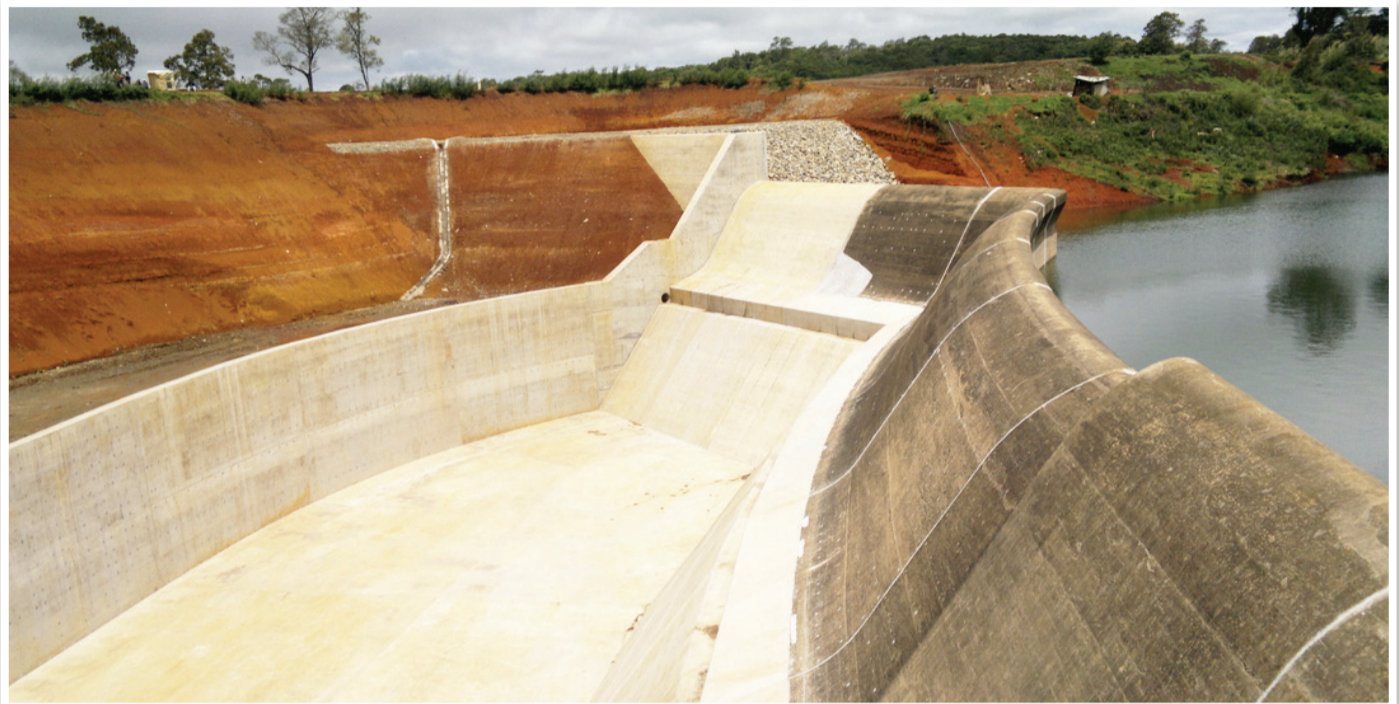
A Section of Sasumua Dam (Spill way)
